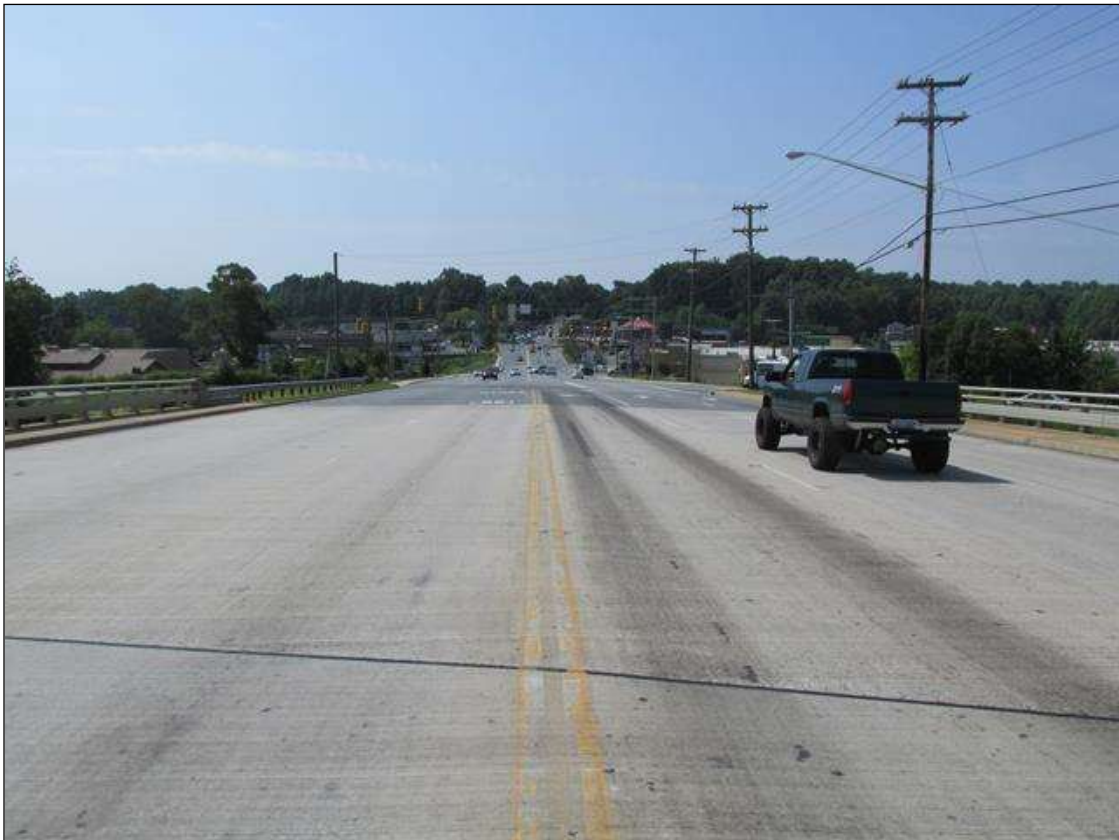
GUARDRAIL LOOKING EAST
