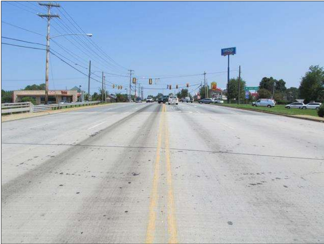
GUARDRAIL LOOKING WEST
