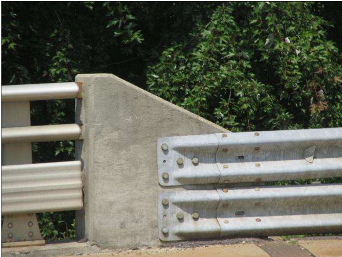
TYP GR CONNECTION FOR SOUTHWEST & NORTHEAST CORNERS
