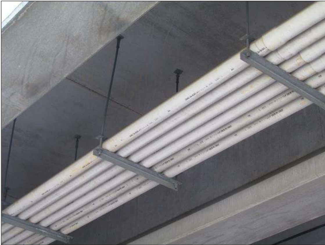
(6) 3" PVC CONDUITS HANGING FROM STEEL SUPPORTS IN BAY 10
